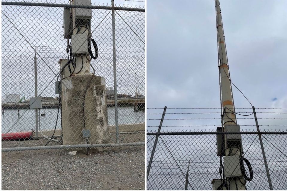
Figure 6: Light Pole (Potential Obstruction) - Howard Terminal
