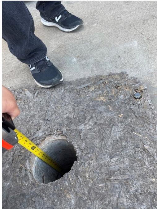
Figure 8: Measurement showing six feet distance between the top sediment layer and top concrete surface - Alameda Site
