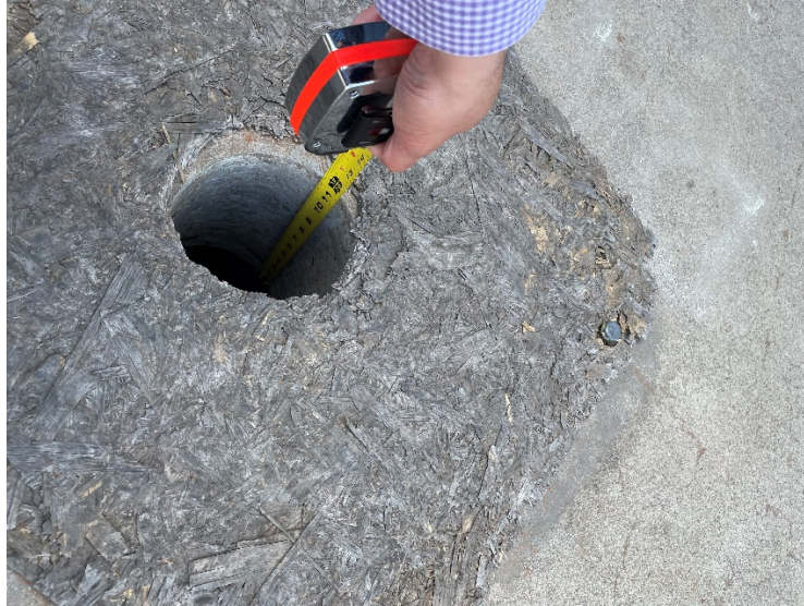
Figure 9: One-foot concrete layer - Alameda Site
