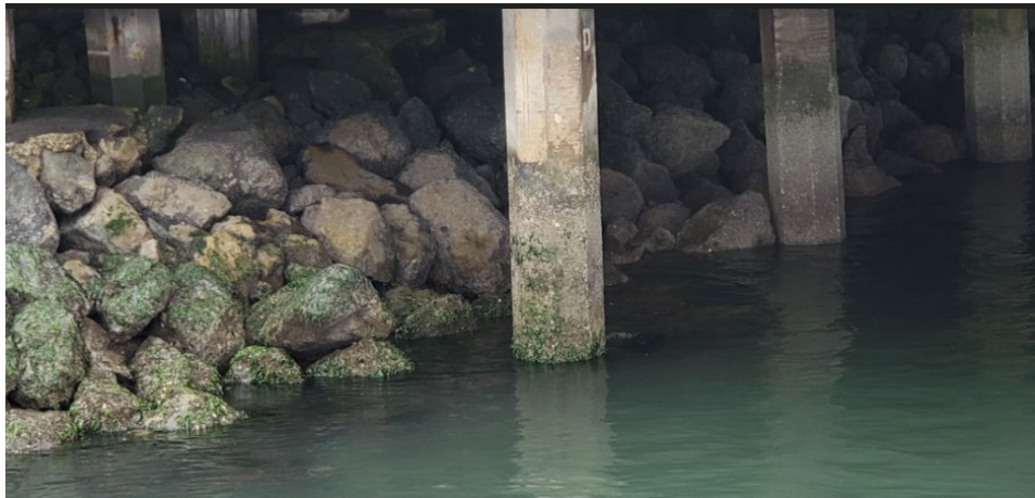
Figure 5: Rip-rap on the Rock Dike - Howard Terminal
